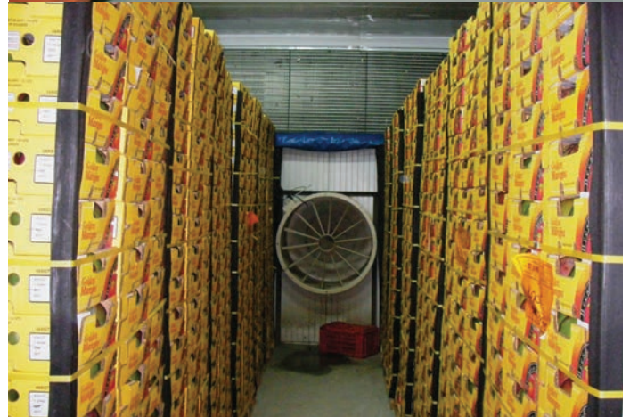
Forced-air cooling tunnels
