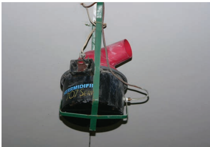
A storage room humidification unit
