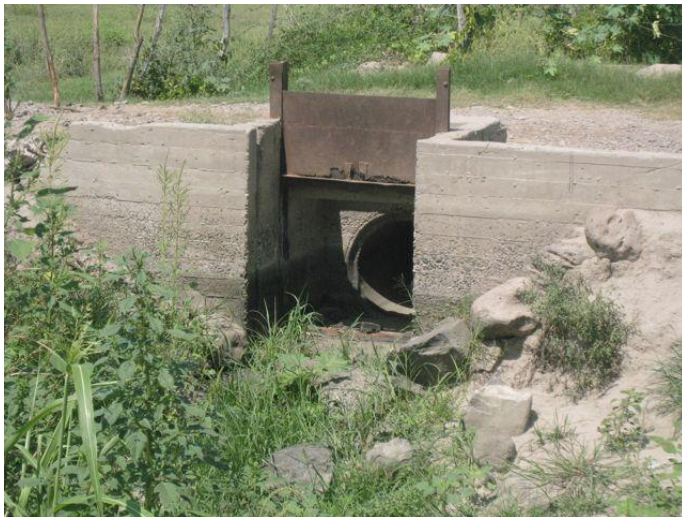
Irrigation ditch to control water within canals
